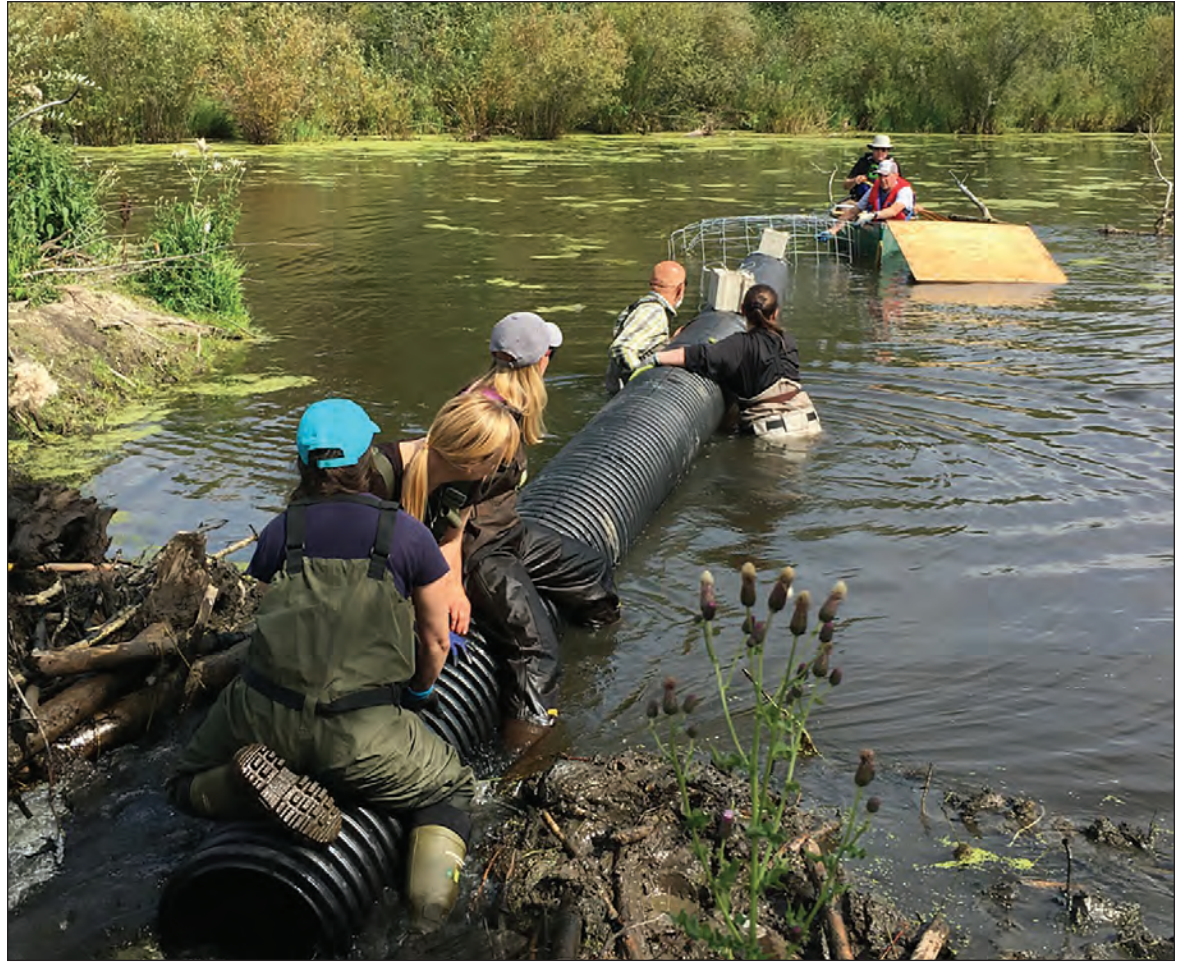
Pond levellers help control the depth of water upstream of a beaver dam to prevent flooding. The pipe lies on the pond floor following installation, which is a team effort. | COWS AND FISH
